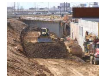
In late-spring construction, excavators build an embankment to support the widened southbound lanes of I-95 between Bleigh Avenue and Cottman Avenue.
