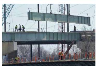
Left: Workers remove a steel girder from the old ramp to I-95 south from Aramingo Avenue.
