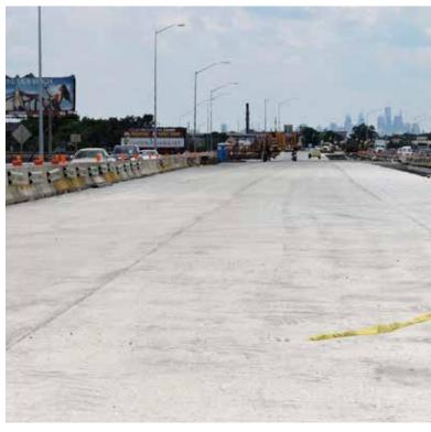
Concrete paving on the widened and rebuilt northbound lanes between the Bridge Street and Cottman Avenue interchanges will wrap up by early fall. Work will then shift to the median.
