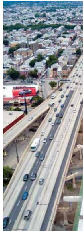
**New concrete pavement for a section of the new northbound I-95 viaduct stretches north from near Girard Avenue to Ann Street and beyond. As the new viaduct finishes in 2018, PennDOT will begin the early stages of replacing the adjacent southbound viaduct. Photo: James J. Anderson Construction**
