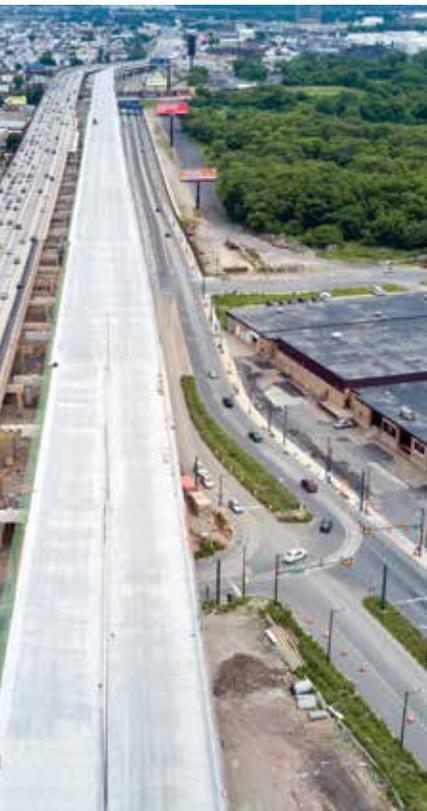
Northbound I-95 traffic exiting at Girard Avenue uses the new off-ramp to Richmond Street as deck construction progresses south toward Palmer Street. (Note the burlap covering recently poured concrete at the bottom of the photo and the as-yet unpaved segment with green re-bars in place.) *Photo: James J. Anderson Construction*
