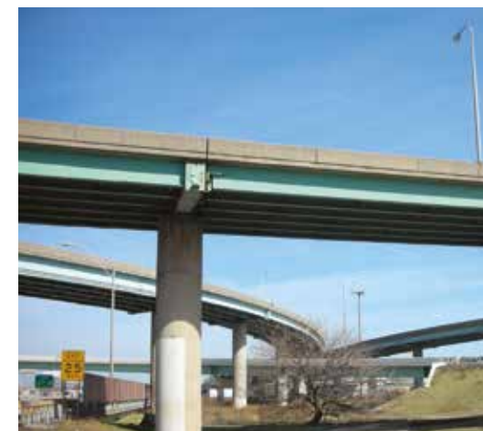
Ramps at the Betsy Ross Bridge Interchange
