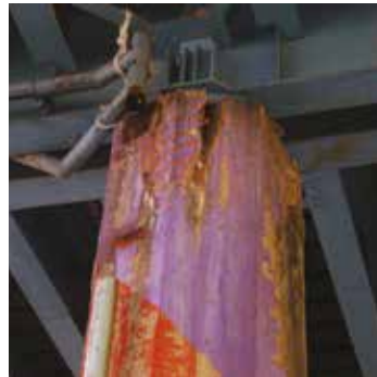
After cracks were found in a column supporting I-95 near Ann Street (left), workers installed a temporary support (right) and replaced the damaged column.
