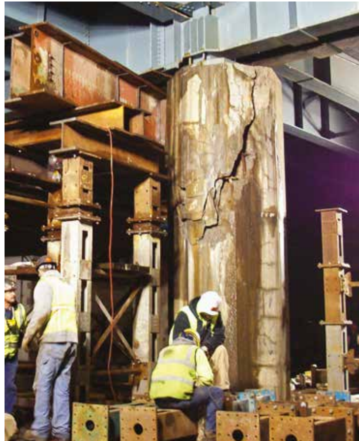
After cracks were found in a column supporting I-95 near Ann Street (left), workers installed a temporary support (right) and replaced the damaged column.
